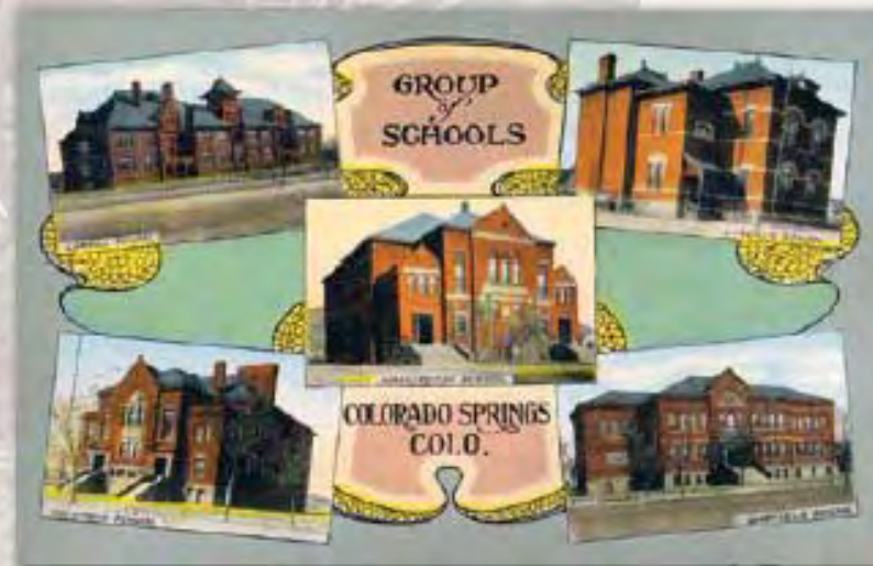
ABOVE Harris financing helped Colorado Springs, Colorado, build its schools in the early 1900s.
